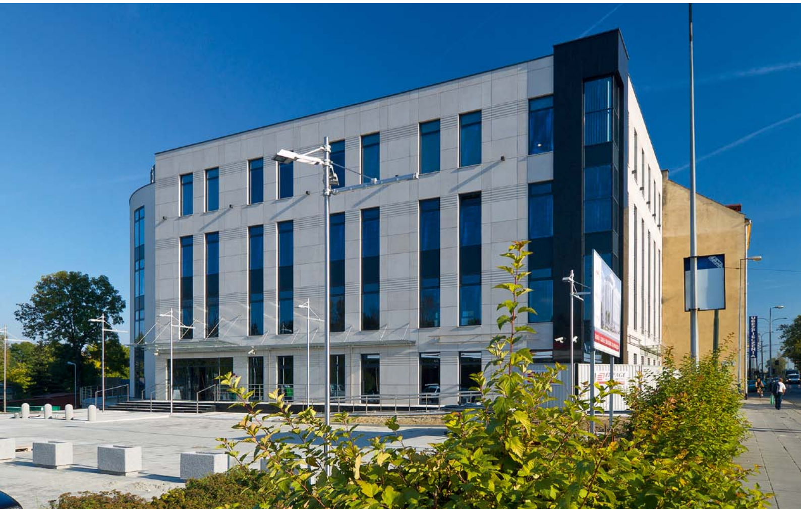
Office building W22 located on 22A Wielicka Str.
