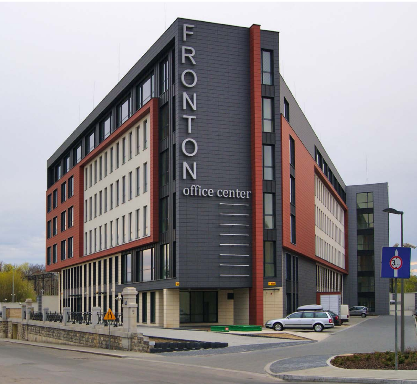
Fronton Office Center
